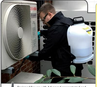
Designed for use with Advanced concentrated and ready-mixed coil cleaner chemicals, both indoors and outdoors. Boasts a capacity of 15 litres, with supportive back pack-style straps. Fully rechargeable battery that supplies the 12V electric sprayer with all its power.
